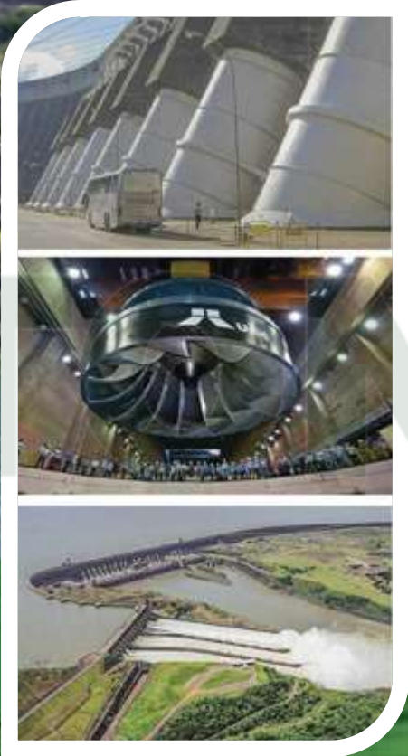
Itaipu Hydroelectric Power Station, Brasil Fire Detection for the world's largest hydroelectric power station
